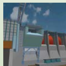
Spillway weirs at Ice Harbor, Lower Granite and Lower Monumental Dams are designed to be 'removable,' by controlled descent to the bottom of the dam forebay. This capability permits the spillway to perform to its original flow
