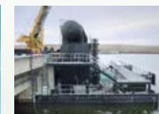
Spillway weirs are mounted onto a dam's forebay where they draw fish toward their smoother water flow over the spillway.
