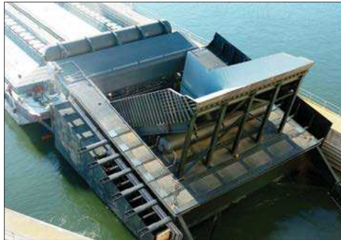
U.S. Army Corps of Engineers Photos
