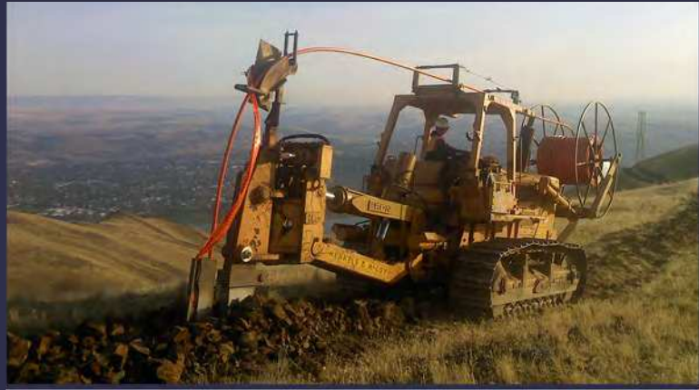
Installing High Speed Internet Infrastructure for Businesses and Residents
